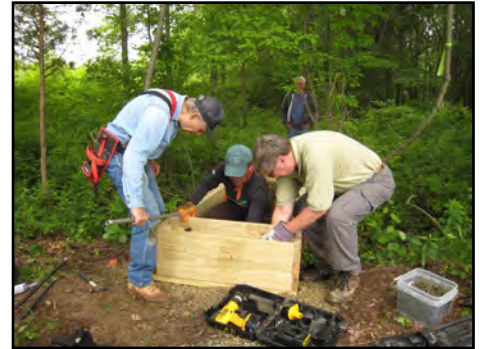
George Solovay (left) and team construct the bridges.
